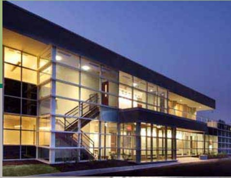
ASHRAE Headquarters - Atlanta, GA
