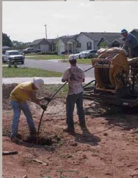
Pipe Loop Insertion
